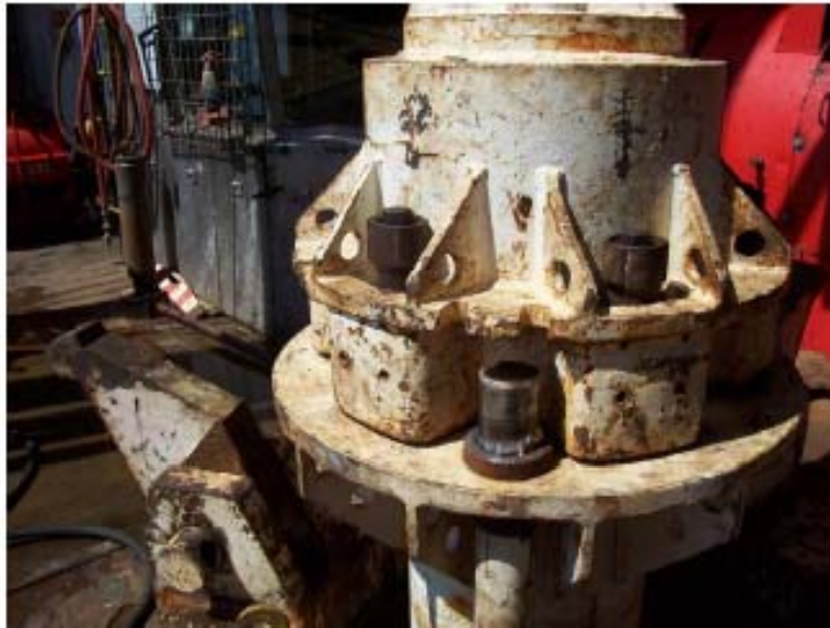
Figure 3. Gap Between FD8 Lift Sub & Riser Pin Flange
