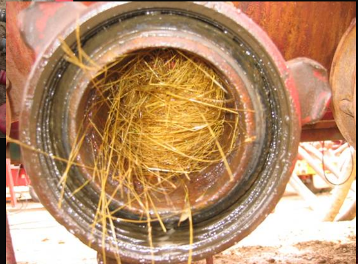
Suction hoses / manifold become blocked
