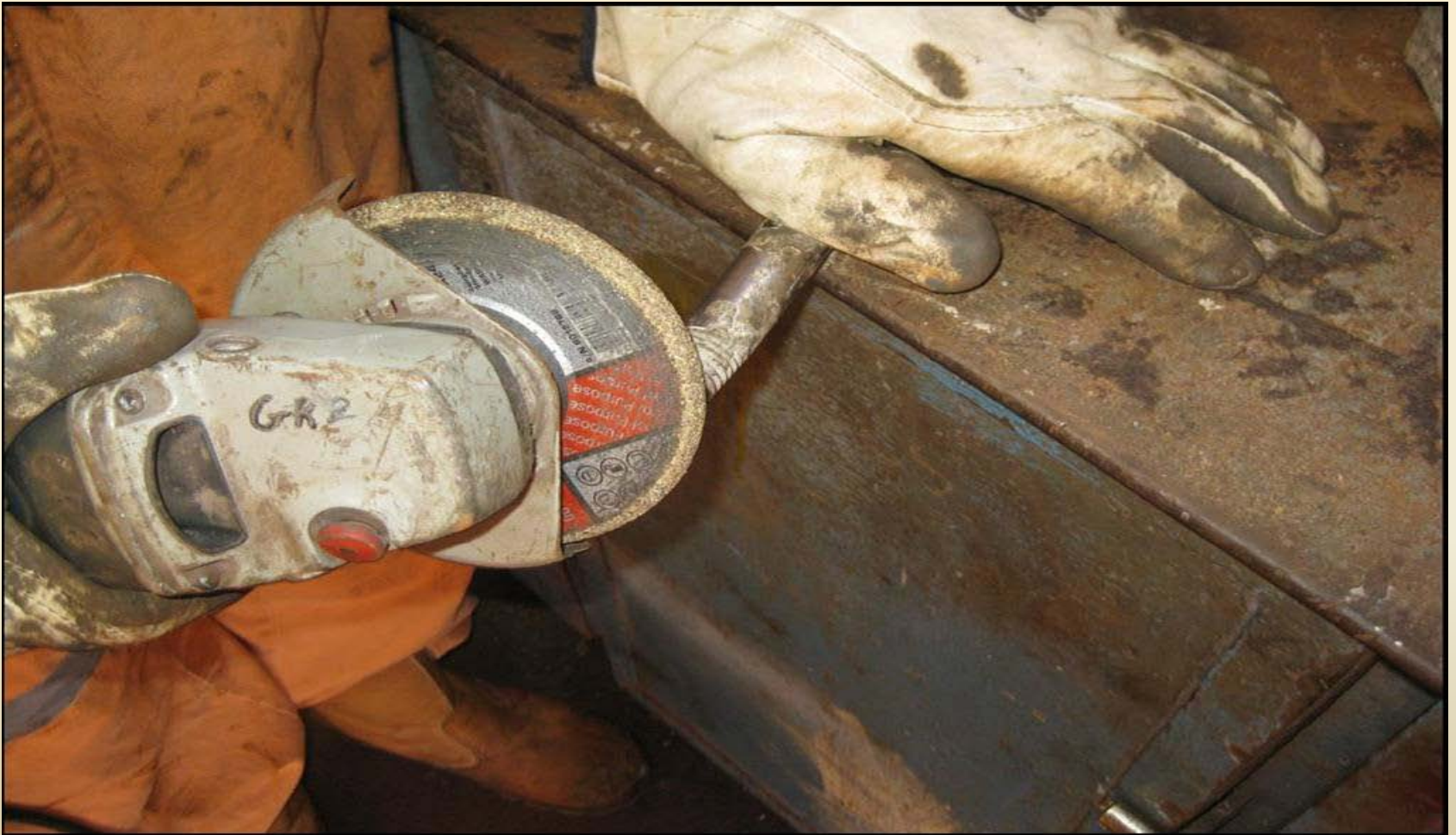
Work Practise being undertaken at the time of the incident
