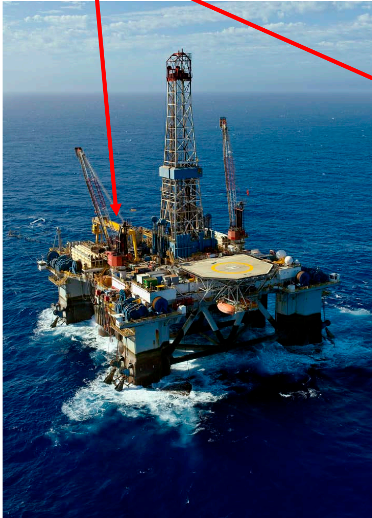
Gantry Crane – Traverses Pipe Deck
