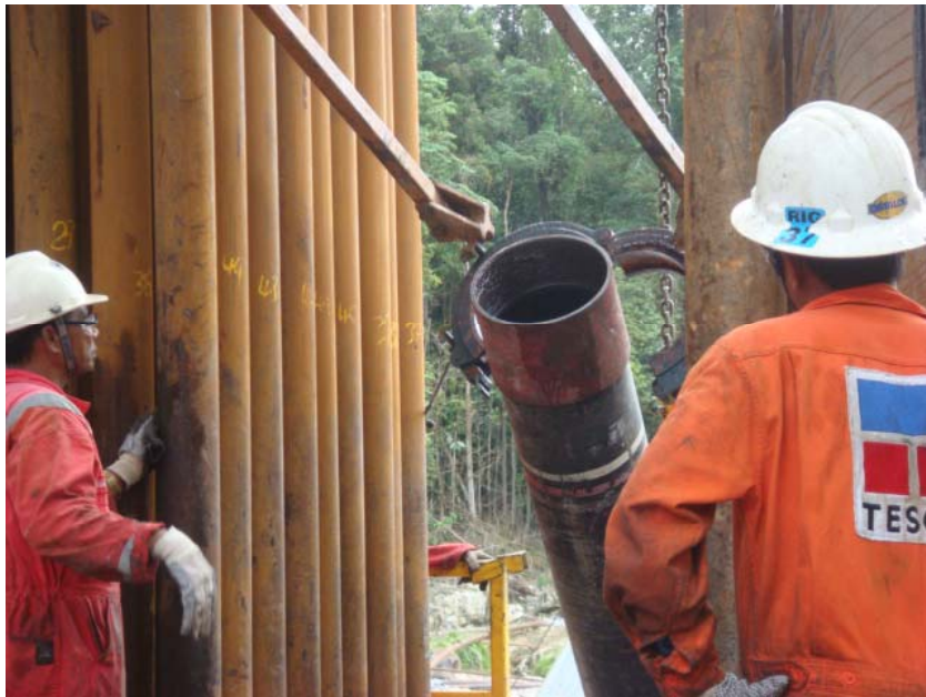
Elevators being latched from above the casing.
