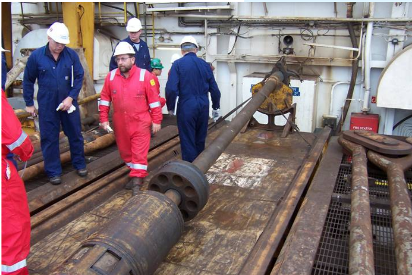
Tool position prior to impact
